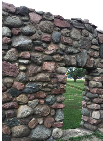
Detail of stone construction in the bandshell entrance.
