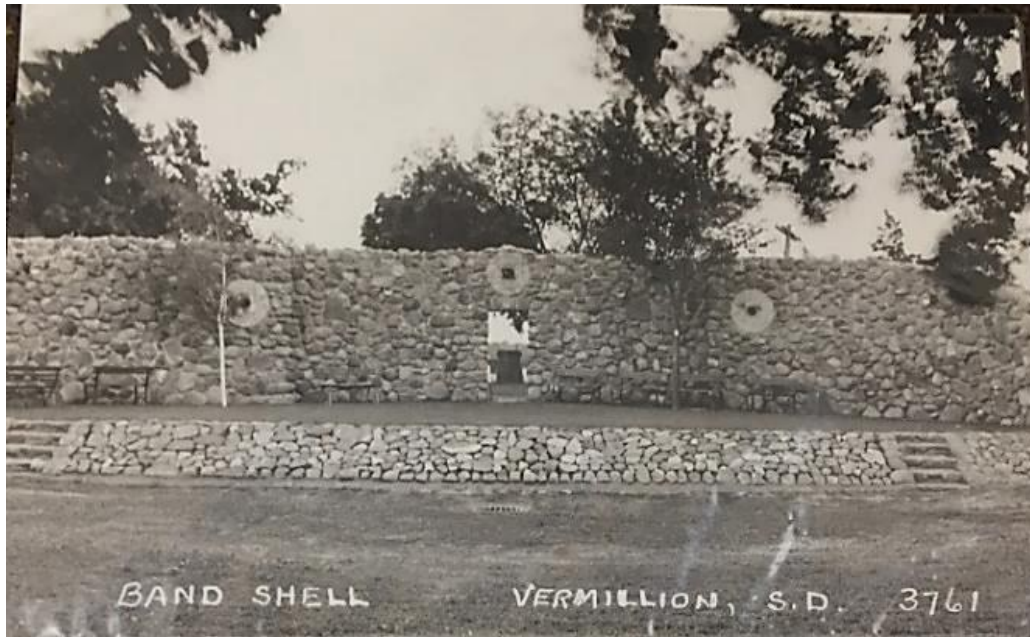
The Prentis Park bandshell with embedded buhrstones (early undated postcard). Note that the front of the stage and the steps on either side of the stage were also constructed of stones.
