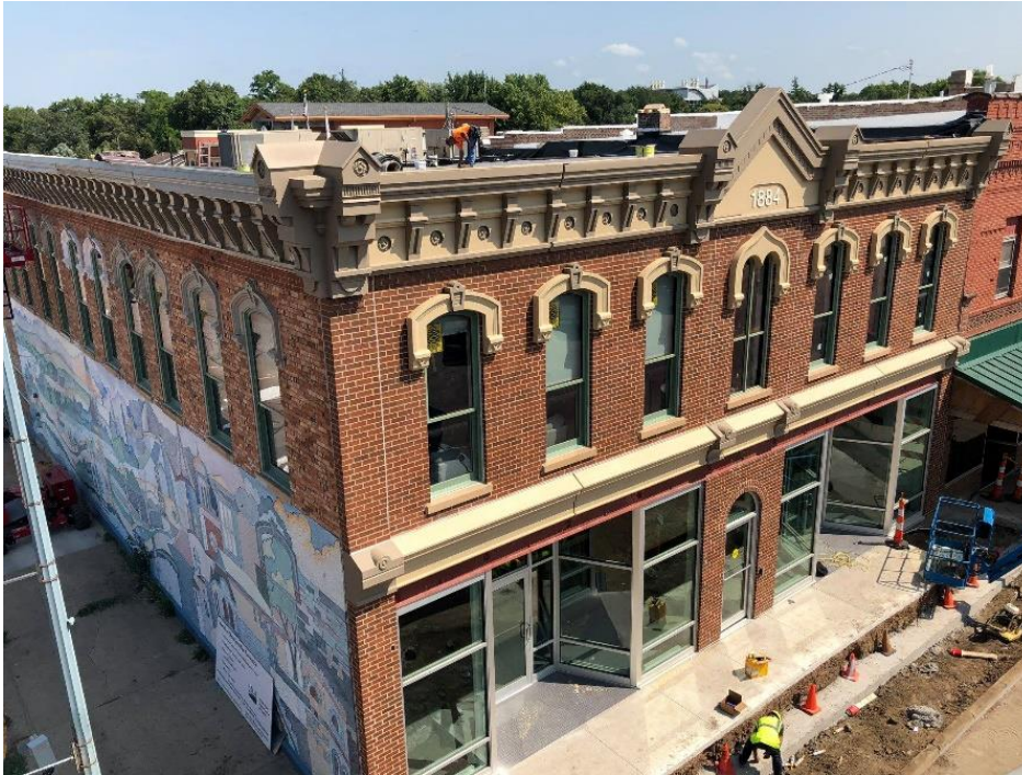
Removal of the façade of the building and replacements to emulate the original structure.
