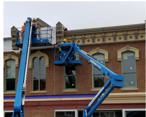
Removal of the façade of the building and replacements to emulate the original structure.
