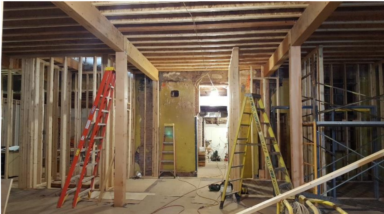
The first and second floors were completely gutted before new walls were framed. The first-floor rear entrance was recreated. Note the brick walls in the back near the door. (VCDC photographs)
