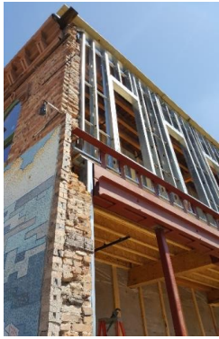
Removal of the façade of the building and replacements to emulate the original structure.
