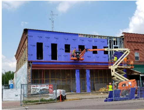
Removal of the façade of the building and replacements to emulate the original structure.
