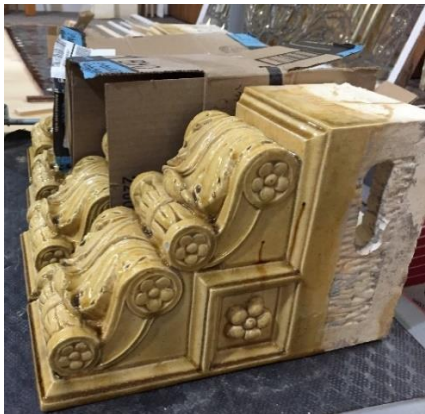
Note the many decorative elements in the cleaned corbels. The unglazed sections were anchored into holes above the fireplace surround tiles.
