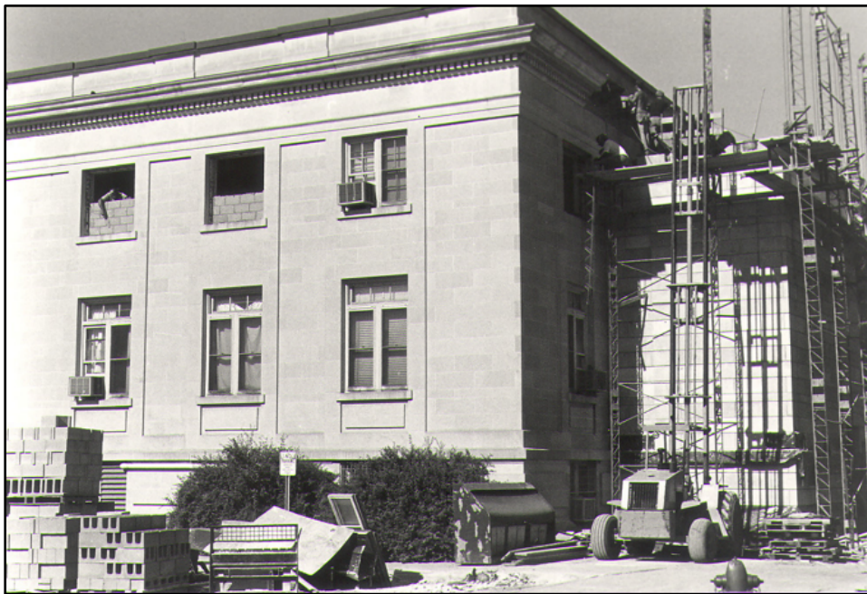
During renovation, windows were enclosed, and an elevator and central air conditioning were installed. Courtesy of Dr. Banks.
