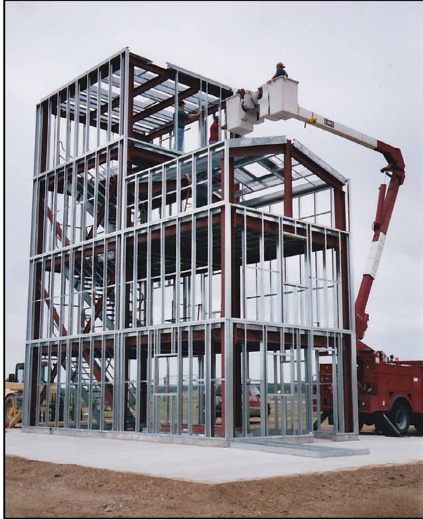
Training Tower July 2005.
