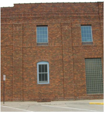
The large window near the front shows the use of glass block as a 1950's treatment to both provide privacy and avoid the purported energy loss and repair problems of regular windows. The second floor windows are modern replacements with fake muntins. The use of brick to produce decorative cornice features and projecting columns breaks up an otherwise bland facade and is a good indication of what an accomplished bricklayer could do.
