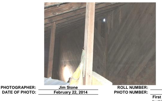
PHOTO NUMBER: First floor, South lean-to, looking NW, 1x8 diagonal sheathing, 4x4 posts supporting 2x6 lean-to rafters.
