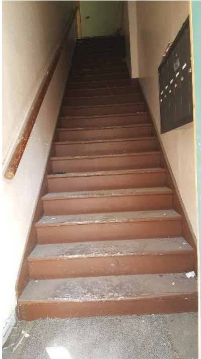
The very steep staircase to the second floor in the east side of the building prior to its removal. Note the mail boxes for upstairs apartments.
