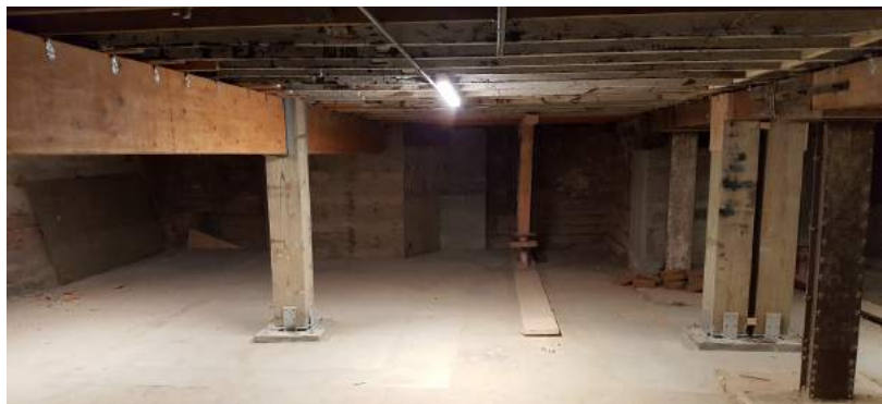
The basement of the building was totally renovated to improve structural integrity.
