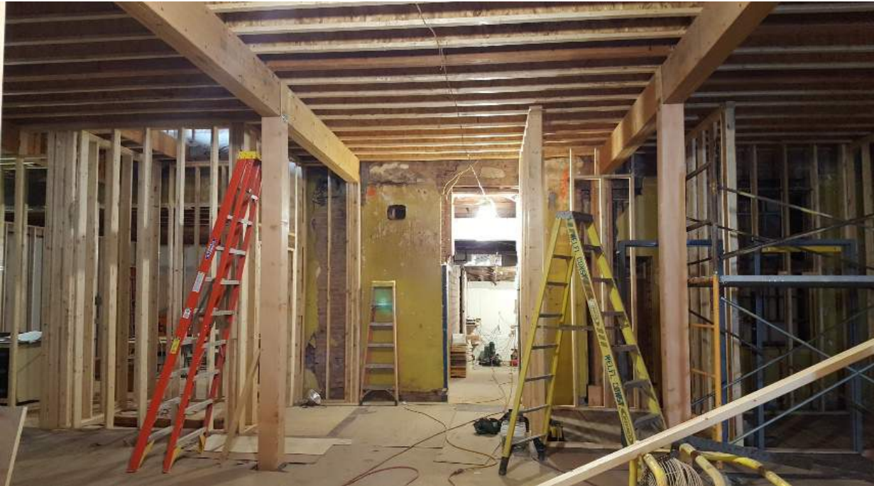
The first and second floors were completely gutted before new walls were framed in. The first-floor back entrance was recreated. Note the brick walls in the back before the door.
