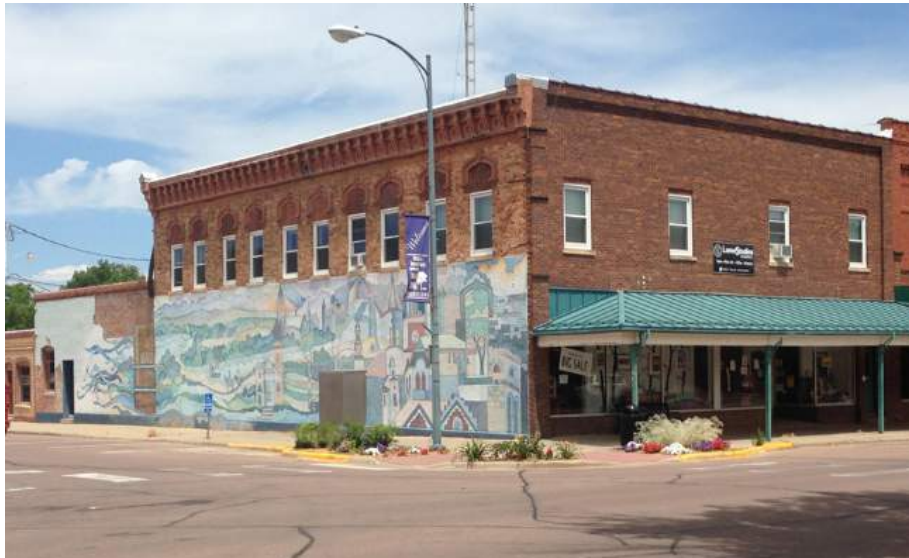
2 East Main during Lumos Studios' occupation of the building, highlighting the Termes mural and buildings connected to the rear of 2 East Main Street. The original cornices around the window on the west side are also evident.
