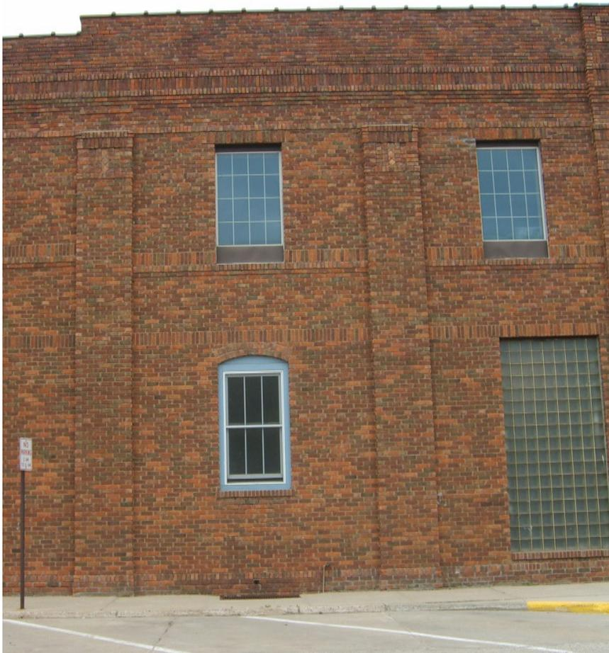
The large window near the front shows the use of glass block as a 1950's treatment to both provide privacy and avoid the purported energy loss and repair problems of regular windows. The second floor windows are modern replacements with fake muntins. The use of brick to produce decorative cornice features and projecting columns breaks up an otherwise bland facade and is a good indication of what an accomplished bricklayer could do.
